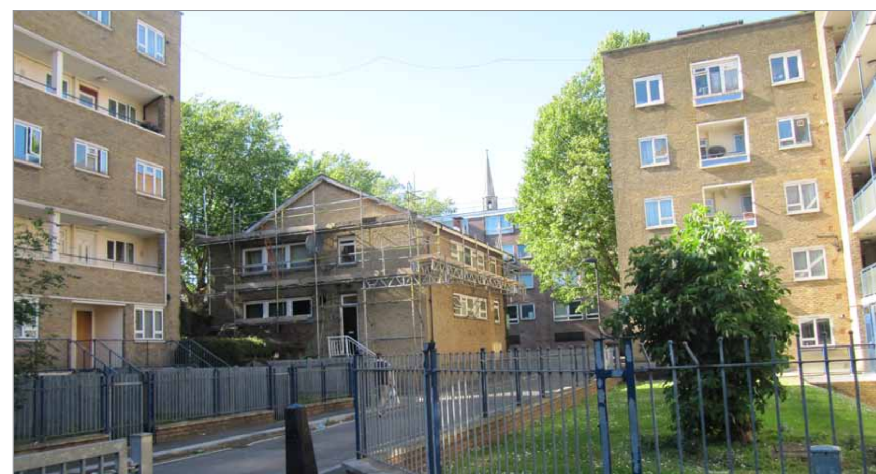
The Victory as seen from Nash Street
